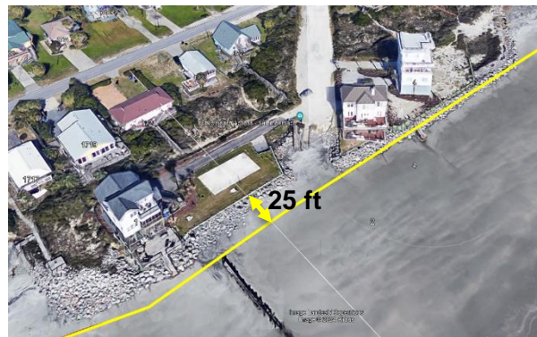
Figure 7. Google Earth image showing that the seawall at Summer Place Lane is set back 25 ft from the yellow PEL/baseline.
